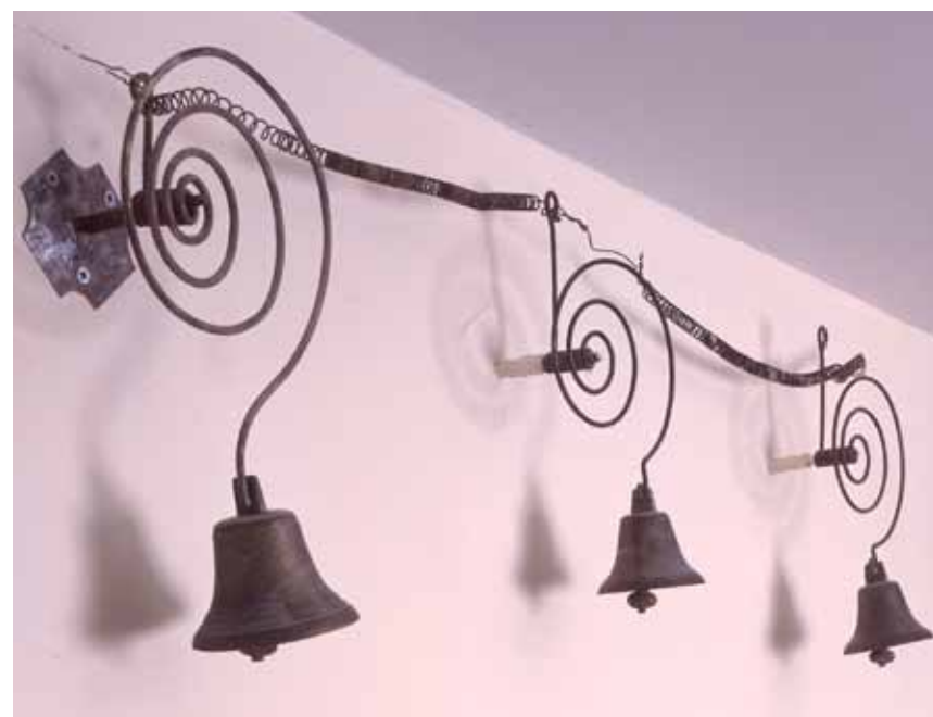
Bells line the kitchen wall at the Merchant's House Museum. Each bell rang with a different note to indicate which room the call came from. The bells were activated by a small lever to the right of the fireplace mantle in each room.
